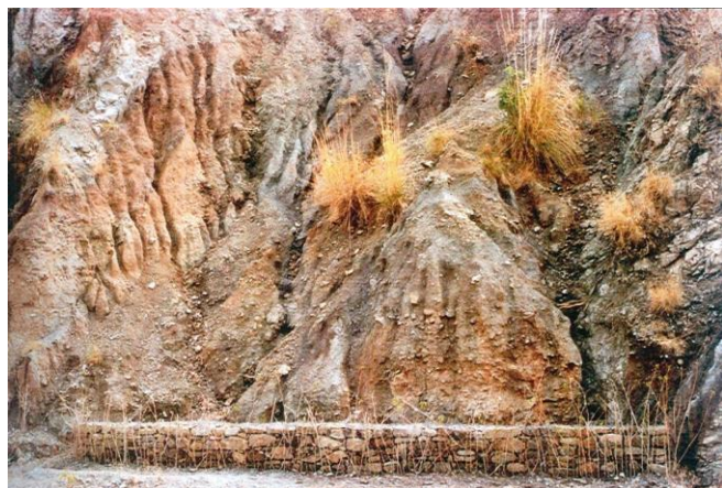
Figure 1 Land degradation problem and constructed gabion wall at Kulahri-Johranpur-Sansiwala watershed (KJS) catchment
