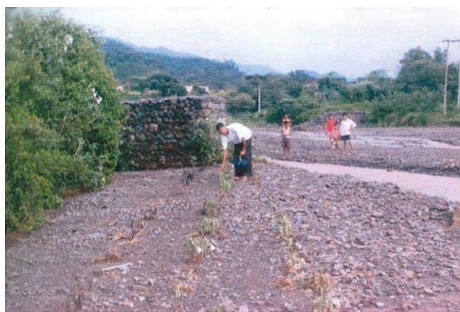
Figure 4 Mechanical and vegetative spurs at downstream of Kulahri-Johranpur-Sansiwala watershed (KJS)
